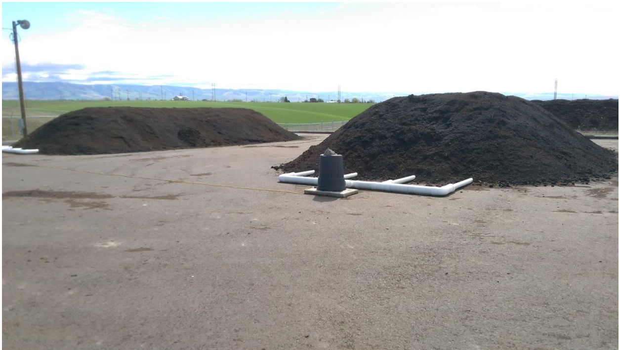
Two Completed ASP's, each ~ 200 Cubic Yards in Volume
