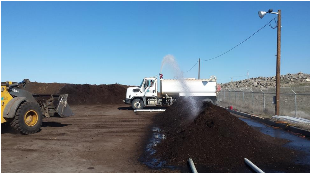
Adding Water (~4,000 gallons) to Moisture Condition the Initial Mix
