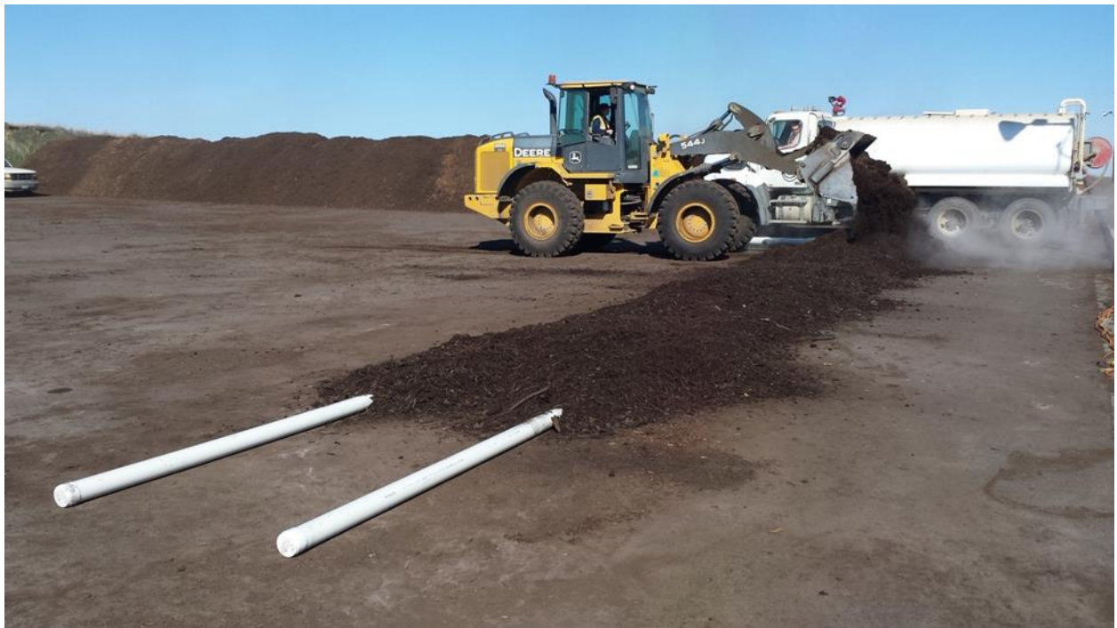
Placing Clean "Screen Overs" as a Plenum Layer on top of the Aeration Pipes
