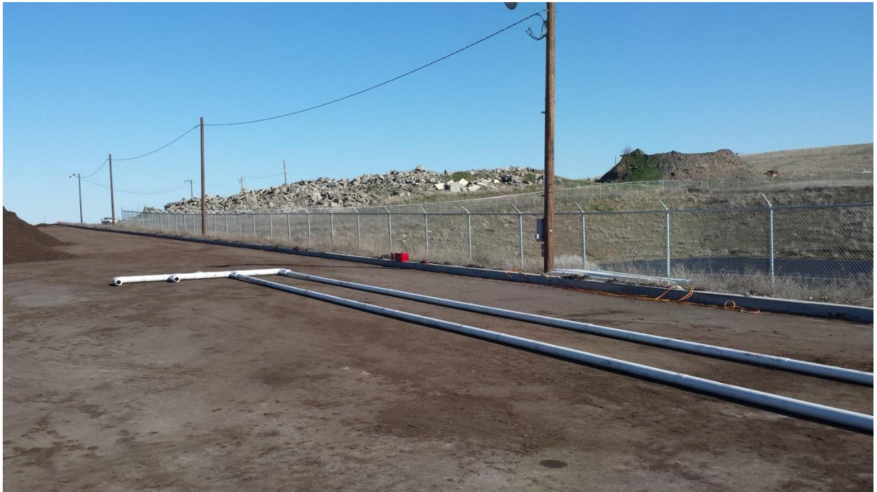
Assembling the 4-Pipe Aeration Manifold and the First Two Lateral Pipes
